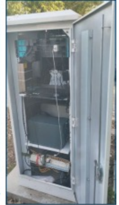
Figure 5. Deployment scenarios of Roadside MEC Equipment (in roadside cabinet).
