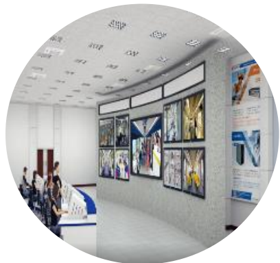
Train Operation Status Monitoring System
